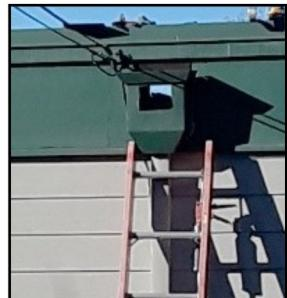
Repairs were made to the roof as a result of leaks we've had in the narthex and the worship supply closet in the back of the sanctuary. This involved resealing downspout scupper boxes. We also had moss removed from the sanctuary roof, and treated it to help prevent moss from coming back.
